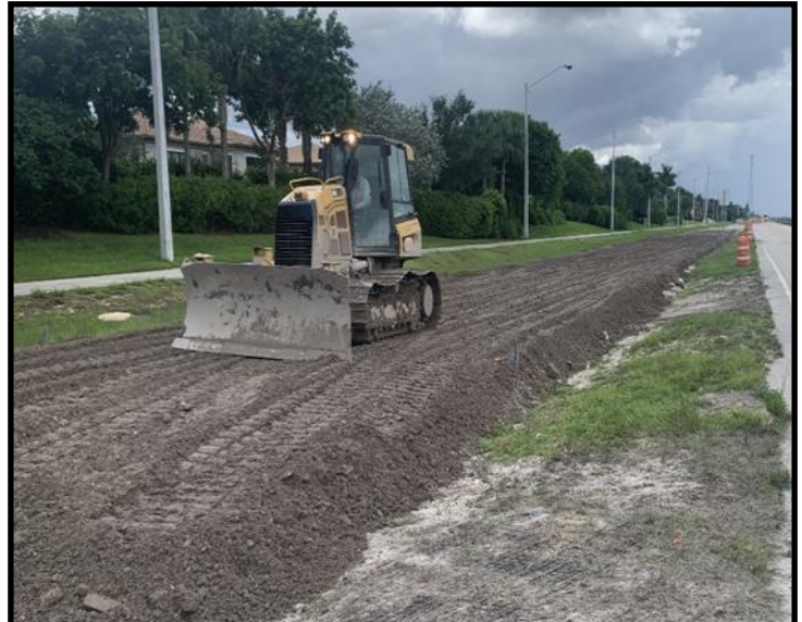
Stable Base Layer Installation for Eastbound Lane
